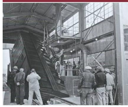
Before we got used to the jumbo covered hopper cars so prevalent now, grain was shipped in a common 40' boxcar. In the early days grain was shipped by the sack. Bulk grain shipment by rail required the use of a temporary grain door secured inside the doorway. In the picture to the left, the wooden door has been removed and the men are manually shoving product out the door.
